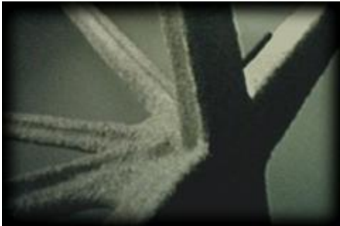
Sprayed-on fireproofing material
